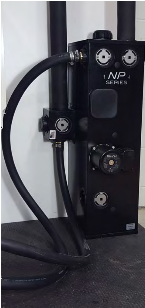
Figure 7: Flow center mounted 3-way valve
