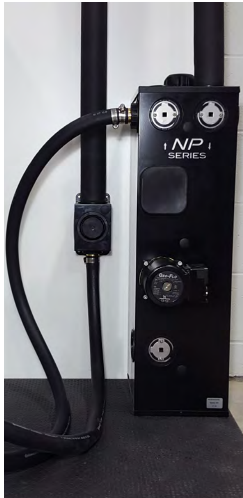
Figure 8: Wall mounted 3-way valve
